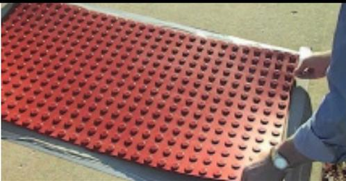
The **Surface Applied** panel is the perfect solution for retrofitting existing concrete surface or new construction, our surface applied detectable warning panels are constructed of an exterior grade, fiberglass polymer composite material.
