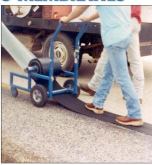
"...waterproofing membranes have reduced the rate of reflective cracking...even when reflective cracking appears over joints with membrane treatment, the cracks appear to stay tighter than cracks over joints without membrane treatment."
